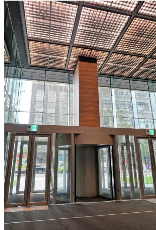
Special revolving door that encloses a building pillar
