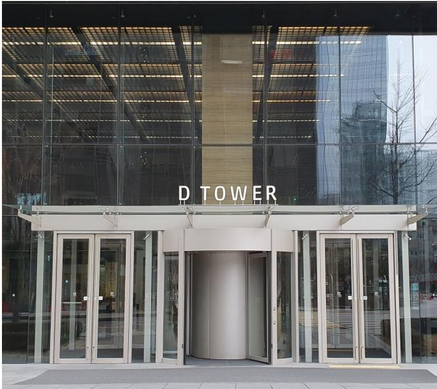
Special revolving door that encloses a building pillar
